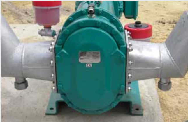
Feed pump for a biogas substrate. Flow rate up to 40 m 3 /h at a pressure of 2 bar.
